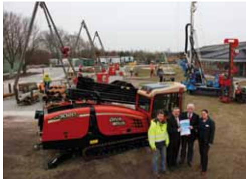
➍ On 7 March 2012, the appointment certificate in accordance with GW 329 was presented to the recognized training Institute BAU-ABC Rostrup in Bad Zwischenahn.
